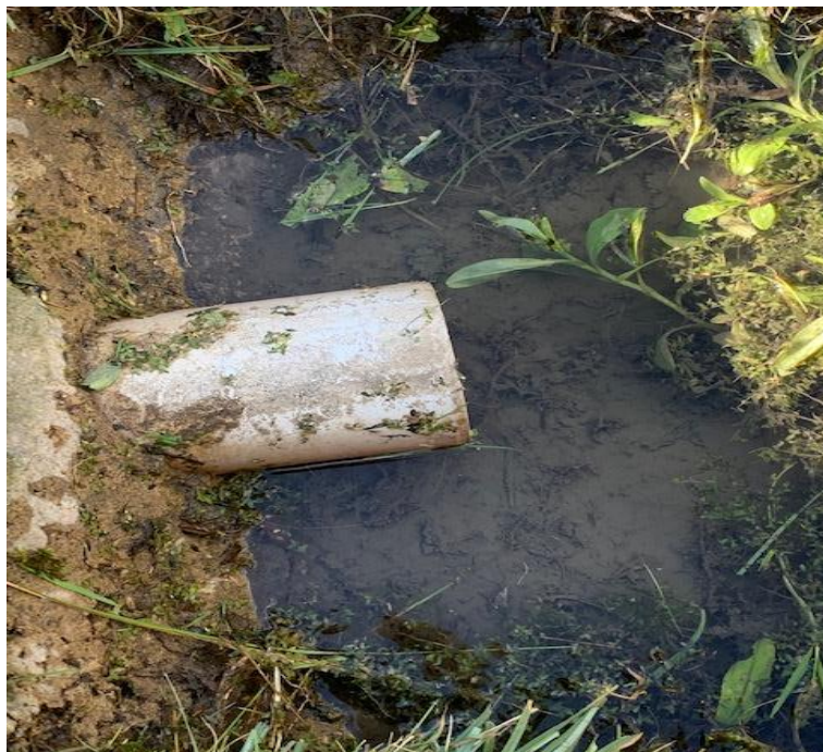
100mm land drain from the playing field, outfalling into Pond D
