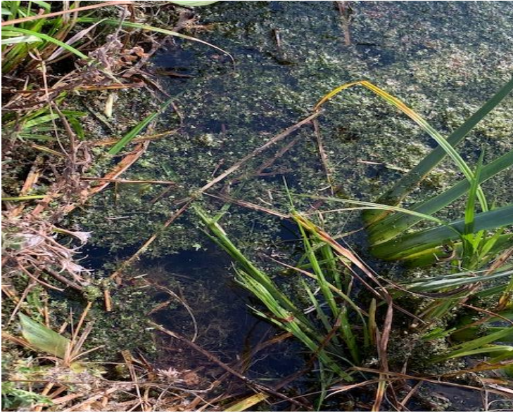
Outlet pipe from Pond D, low level. Bottom photo shows low level pipe inlet to Pond E.
