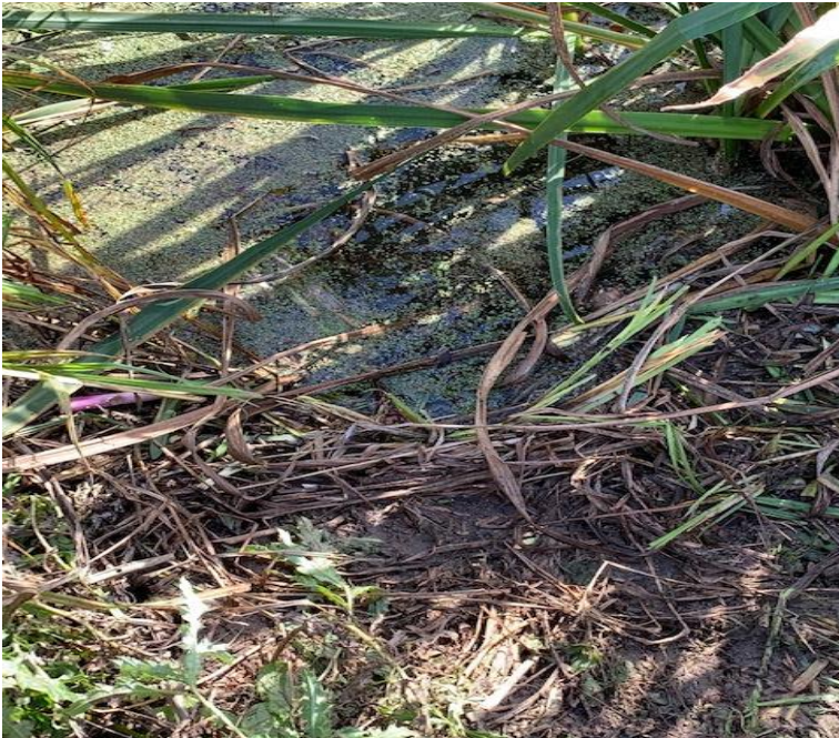
Location of inlet pipe to Pond C, low level connection
