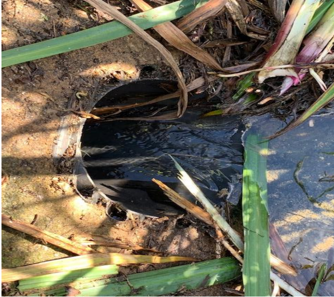
Pipe outlet from Pond E
